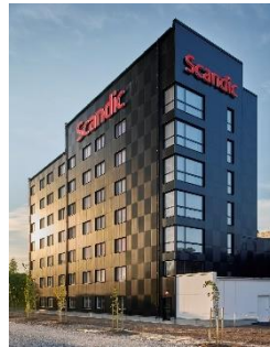
Scandic Luleå Property Management Extension of 117 rooms, F&B, meeting areas Completed Q4 2021 Investment: MSEK 154
